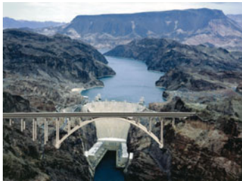
Hoover Dam, with recently completed Colorado river bridge
